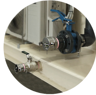
Interconnection provisional flanges for rapid set-up
